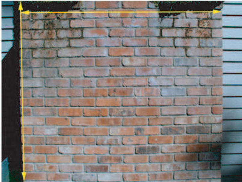
Figure 3.2: Using wide angle lenses recognizable lens distortion occurs. Straight lines become curved.
